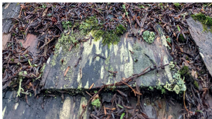
The deteriorated cedar shingles
