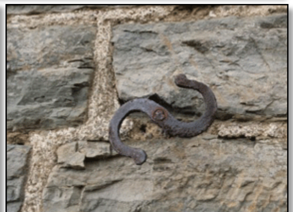
Original fitting and mortar on south wall
