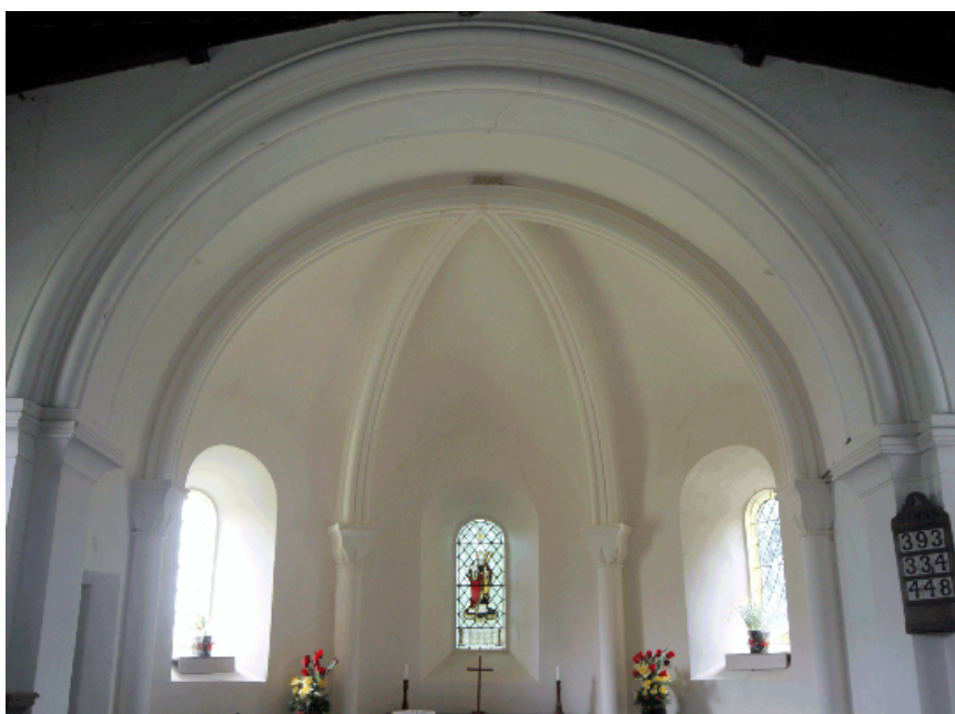
Ribbed and Vaulted Apse
